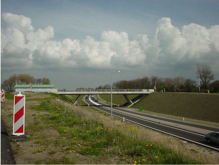
Figure 8.15: Brand new overpass over the N99 at Westerland, the Netherlands. Photo by Jan-Simon Hoogschagen (from http://www.pagowirensse.nl/ ).
