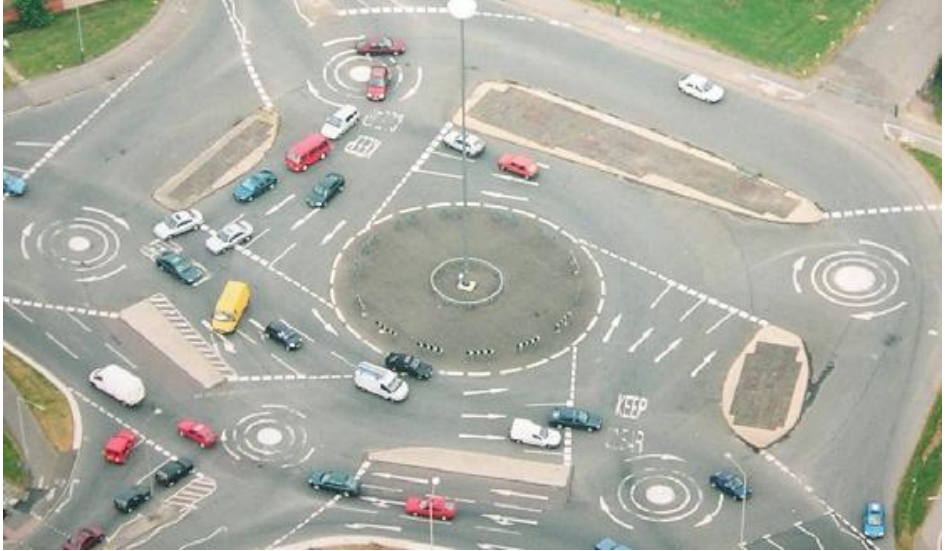
Figure 8.8: Swindon, UK, has what they call a ‘magic roundabout’ with both clockwise and counter-clockwise rotation. Image from http://p.vtourist.com . See http://tinyurl.com/yerfon for a google satellite view.
